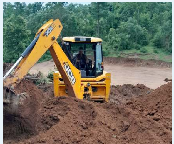
Progress of the community hall at Pdieniadaw village, Thadlaskein Block
