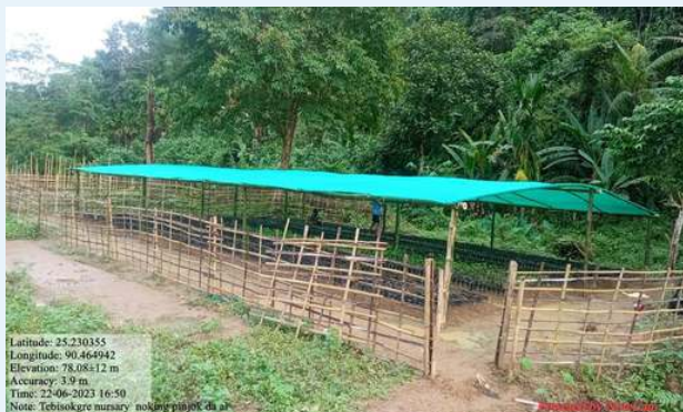
Tebisokgre village completed repairing their damaged nursery due to wind
