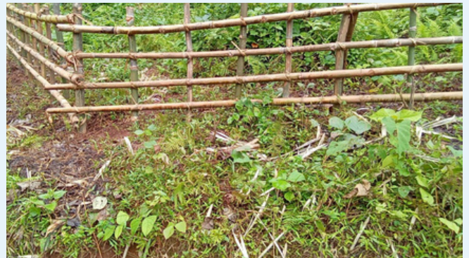
Fencing completed in Gambil Apal village.
