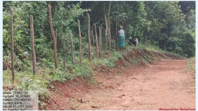
Fence poles have been erected in Derikgre
