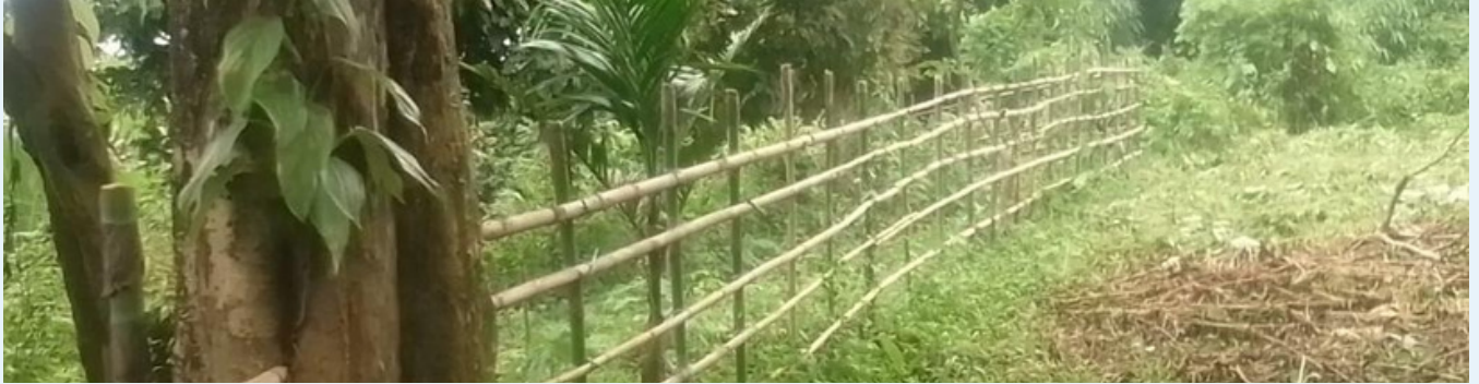
Fencing completed in Songmagiri village on August 11, 2023.
