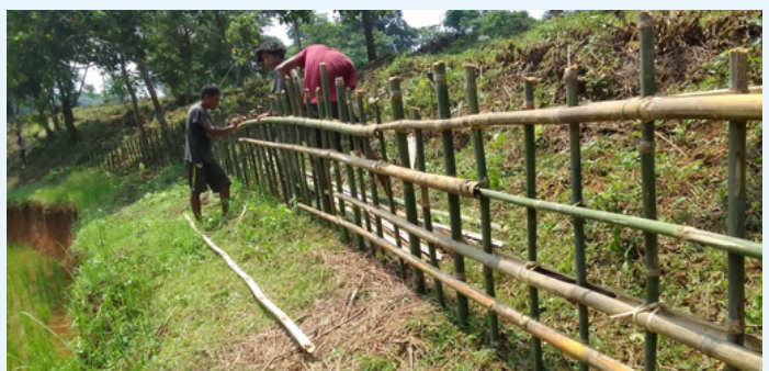
Fencing at Ajasiram village.
