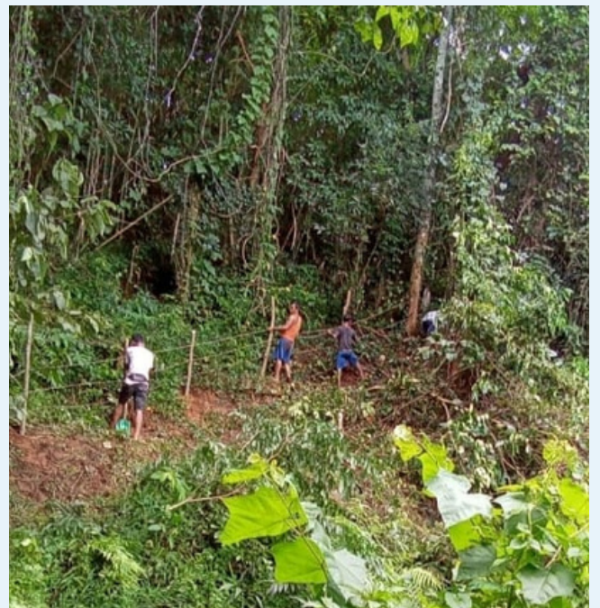
Fencing work at Renchagre village.
