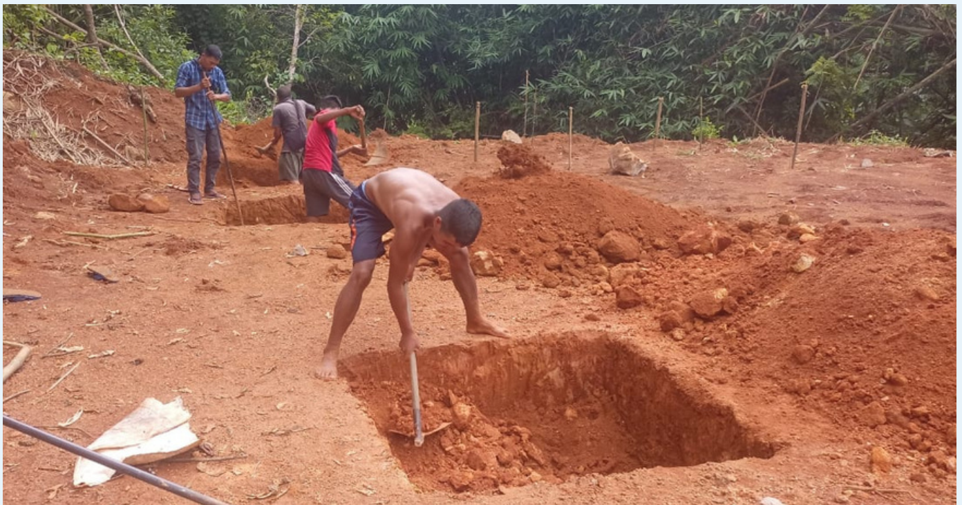
Earthwork in excavation of footing at Bleishiah village.
