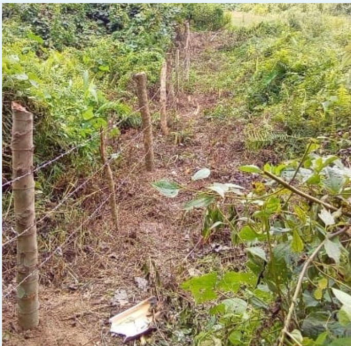
Fencing work at Anogre village.
