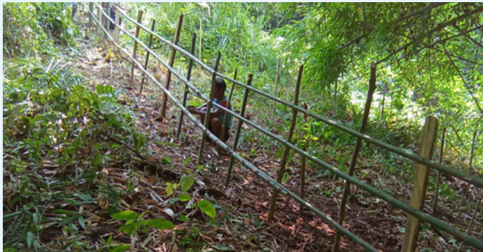
Fencing in progress in Dambo-Chare village.
